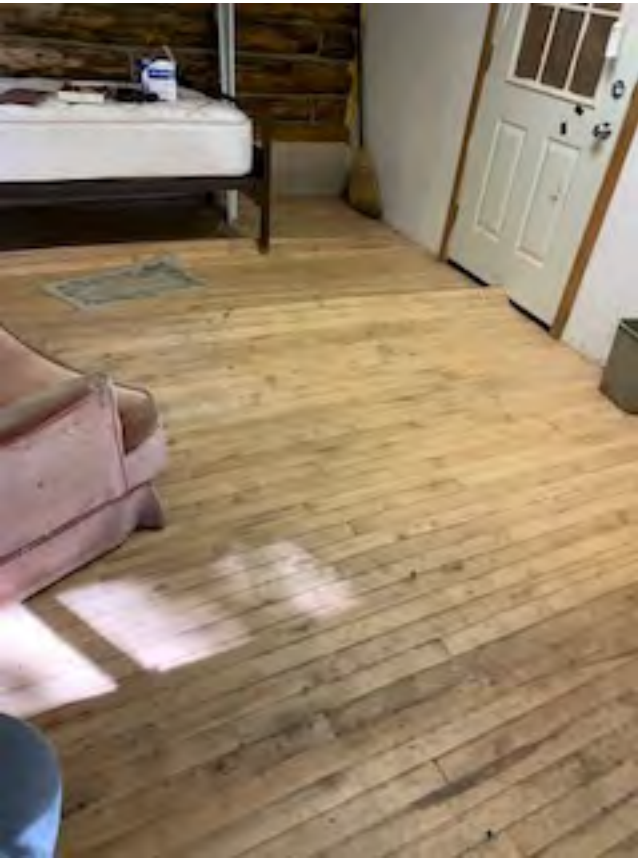
Tile floor cabin
